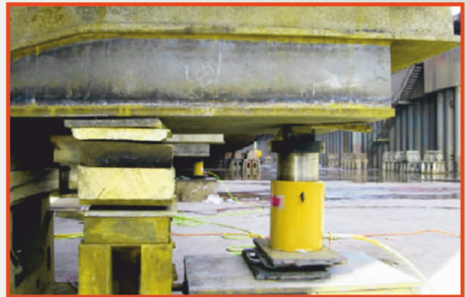
Eight ALSG-2506 cylinders equipped with tilting saddles lifted the planking of the bridge as the pier heads were being rebuilt.
